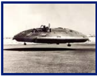
With the termination of the Arrow programme, Avro was left with few contracts. One was for the Avrocar, a vertical take-off and landing circular-wing air-cushion vehicle. A United States Air force funded project, it too was cancelled in 1961 after ten unsuccessful years of research and development. 77
