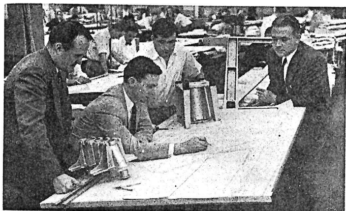
PUTTING IDEAS and problems solutions into readable drawing form is the job of the design office. Here, left to right, Frank Graham, Alan Buley, Bill Bates and Dan Cook consider the redesign of equipment at the wooden mockup stage.
