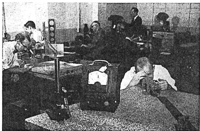
IN STANDARDS ROOM gauges used in the plant or let out to sub-contractors are checked to fractions of a thousandth part of an inch. In foreground working on surface plates are Howard Derouin (left), Cyril Moore. Room is kept at 68 deg.
