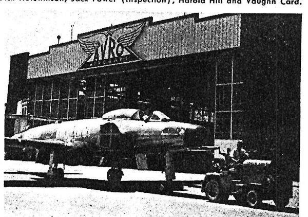
THE BIG MOMENT is when the doors of Bay 3 open and out goes another CF-100 to the flight line for engine and control tests.
