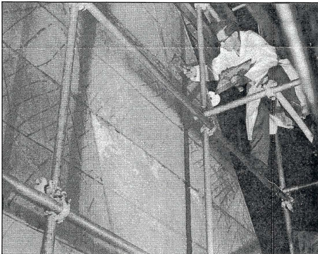
Technician applying phenolic plastic between the templates of the rigs to within one-eighth of an inch of edges, giving a solid core for the plaster finish coat which is treated against moisture.
