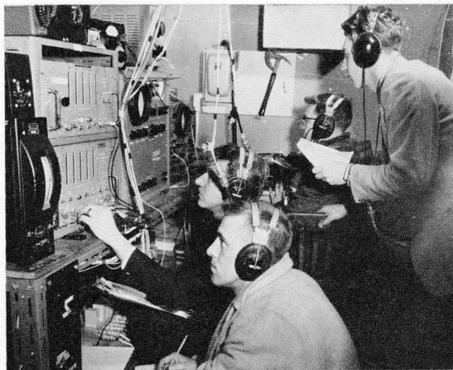
HEAVILY-INSTRUMENTED ARROW transmitted signals to Telemetry Van, above, where complex electronic equipment makes engineering analysis of performance possible while aircraft is still airborne. Operators shown are: Bill Moore, Ray Gibson, Al Maddock and John Lockyer.
