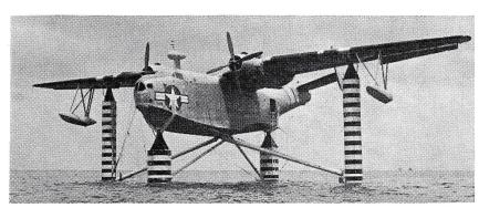
STILT-LIKE VERTICAL FLOATS designed by Convair give this USN PBM-5 a smooth ride on the open sea. The experimental floats provide capability to float on station in open waters with minimum of motion, thereby making a seaplane a stable, working platform for ASW operations. During tests, PBM with vertical floats showed little motion in 4-5 ft, waves, while conventional PBM rocked so violently crew was unable to perform routine tasks.
