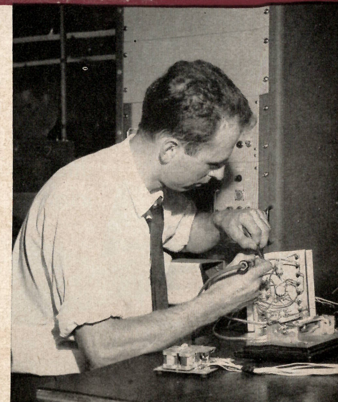
LIFE OR DEATH OF AN IDEA is decided on the testing bench. Bob Johnstone, electrical technician, prepares a breadboard circuit to put a proposed servo system for the Mach Indicator through its paces ... many other tests are to follow.
