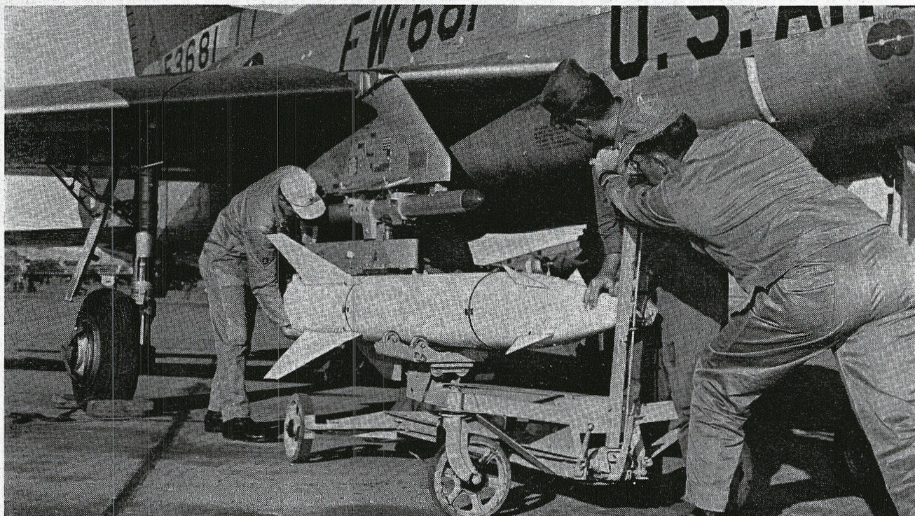
PUGNACIOUS PUP. The addition of this Martin Bullpup to a USAF Super Sabre transforms the fighter into a formidable and accurate bomber, capable of striking tactical targets from outside the range of defensive ground fire.
