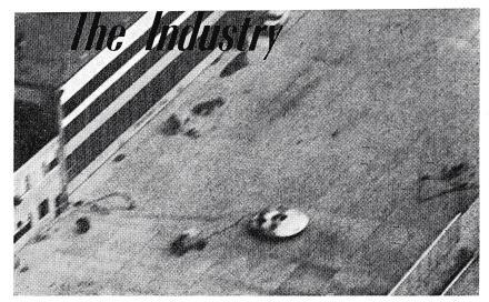
**AVROCAR VTOL AIRCRAFT WAS PHOTOGRAPHED** recently by CBC photographer Jack Judges. Several tethered flights have been made by the Avrocar, which appears to be about 25 ft. in diameter. Opening at centre is probably the air intake. The Avrocar's test pilot is W. J. (Spud) Potocki.
