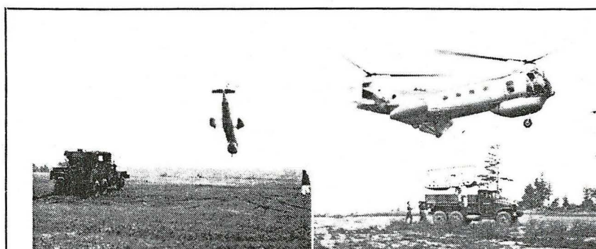
VERTOL 44 DEMONSTRATED: Vertol Aircraft Co. (Canada) Ltd., recently demonstrated a float-equipped Vertol 44 transport to representatives of the armed forces. Left: Helicopter tows an Army M-62 medium 17-ton truck wrecker out of the mud. Right: Precision drop of a two-piece articulated light snow tractor (Rat) onto back of stake truck.
