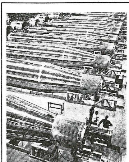
ATLAS ICBM PRODUCTION: First photo of the USAF's Atlas missile production line shows the assembly and check-out section of the line. The stainless steel missiles are 10 ft. in diameter, 75 ft. long. At upper left, booster sections are pulled back to permit installation of boosters and sustainer engine of the Atlas.
