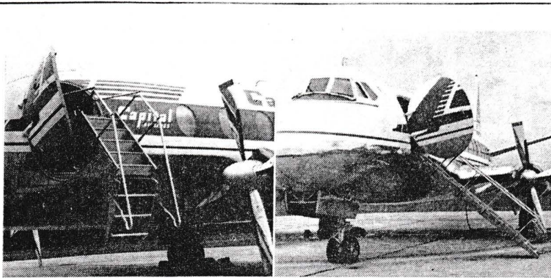
VISCOUNT STOWAWAY: Now available as optional equipment on production Viscounts are these folding passenger stairs, shown here fitted to one of Capital Airline's aircraft. Similar stairs will be standard equipment on the new Vanguard. Vickers-Armstrongs says this is the first time such an installation has been built into a British airplane. Such integral stairs are said to save turnaround time and also to make the aircraft independent of expensive ground equipment.
