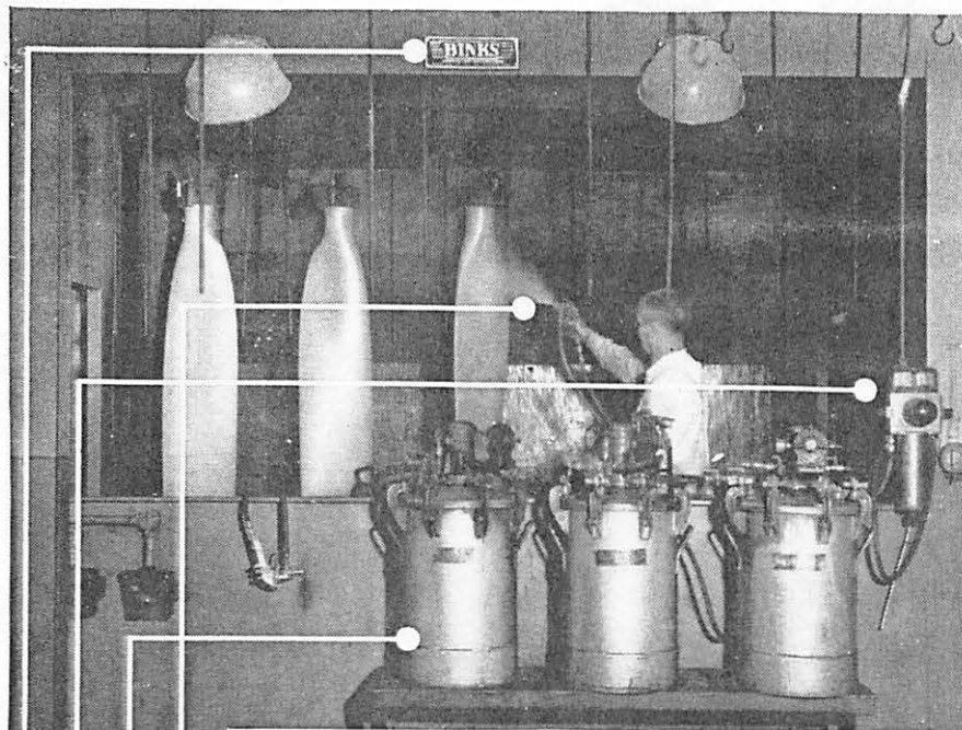
Binks conveyorized spray painting system at a naval air station
