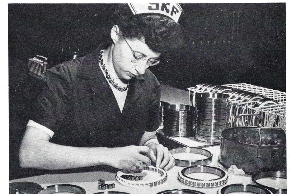
Prototype aircraft roller bearing is being assembled here. Operator places rollers in silver-plated bronze cage before positioning inner and outer rollers.
