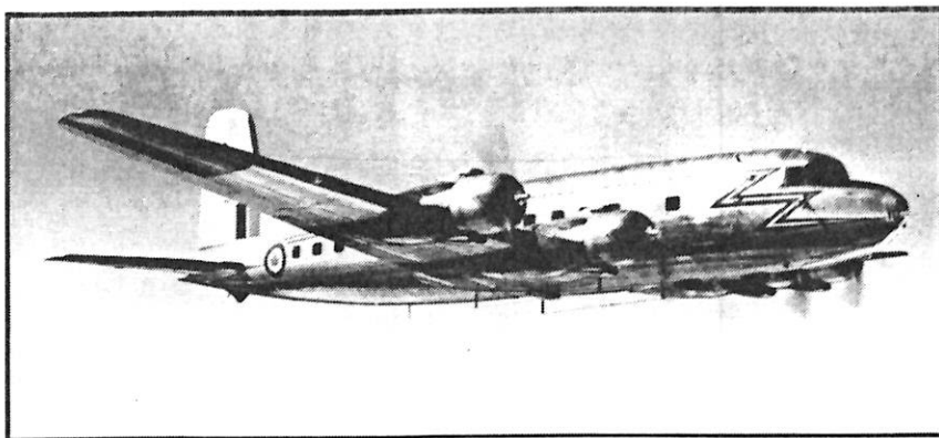
CANADAIR C-5 , only animal of its kind in the world, is basically a North Star re-engineered to take Pratt & Whitney Wasps. It is used for VIP transport.
