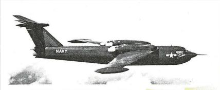
SWEPT, DROOPED, AND POINTED: The USN's new Martin XP6M-1 SeaMaster, which has been undergoing test flying since last July, is described as being "unusually promising". Designed for minelaying and photo-reconnaissance, the aircraft can carry a 30,000 lb. payload and is fitted with a watertight version of the Martin-developed rotary bomb door. The SeaMaster is powered by four Allison J-71A4 turbojets which, with afterburner, each give 13,000 lb. thrust for take-off.
