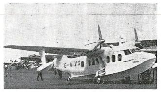
The Short Sealand II is a 5-8 passenger amphibian powered by two Alvis Leonides engines of 520 hp each. BSAA has ordered several of these.
