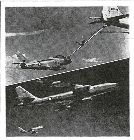
FIRST LINE: Top photo shows an F-86 Sabre being refuelled by a Boeing aerial tanker fitted with a flying boom. Lower picture shows the USAF's first line fighter and bomber team, shown together in flight for the first time. Similarity of lines is interesting. Both aircraft are powered by General Electric J-47 gas turbines, though the B-47 has six as compared to the F-86's one. Both aircraft are in 600 mph class.
