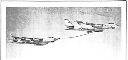
JET TANKER: The world's first jet propelled aerial tanker airplane, the Boeing KB-47B Stratojet, is shown here refueling a B-47 bomber version of the Stratojet. The KB-47B is fitted with Flight Refueling Incorporated's probe & drogue refueling system. The jet tanker was developed by Boeing Airplane Company working in conjunction with the USAF Air Research & Development Command and Flight Refueling.
