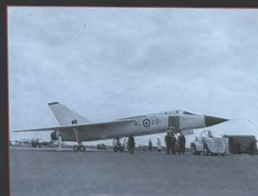
Avro Arrow 25201 showing anhedral of the wing, allowing a shorter landing gear to be fitted.
