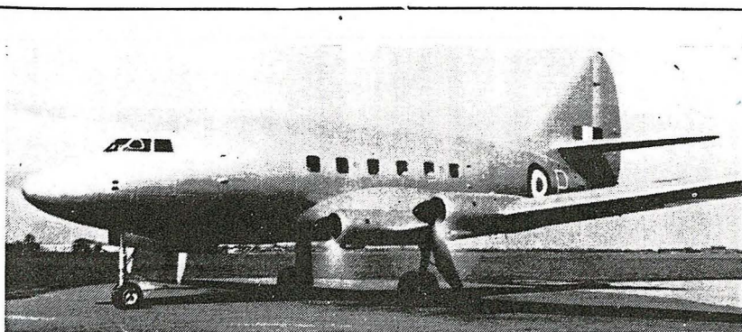
A.W.A. APOLLO: The Armstrong Whitworth Apollo recently flew for the first time in Britain. It is an all metal, low wing aircraft with a laden weight of approximately 39,500 pounds. It can accommodate a maximum of 31 passengers and 7,500 pounds of freight in its pressurized cabin. Power by four Armstrong-Siddeley Mamba II gas turbines driving fully feathering reversible pitch propellers.
