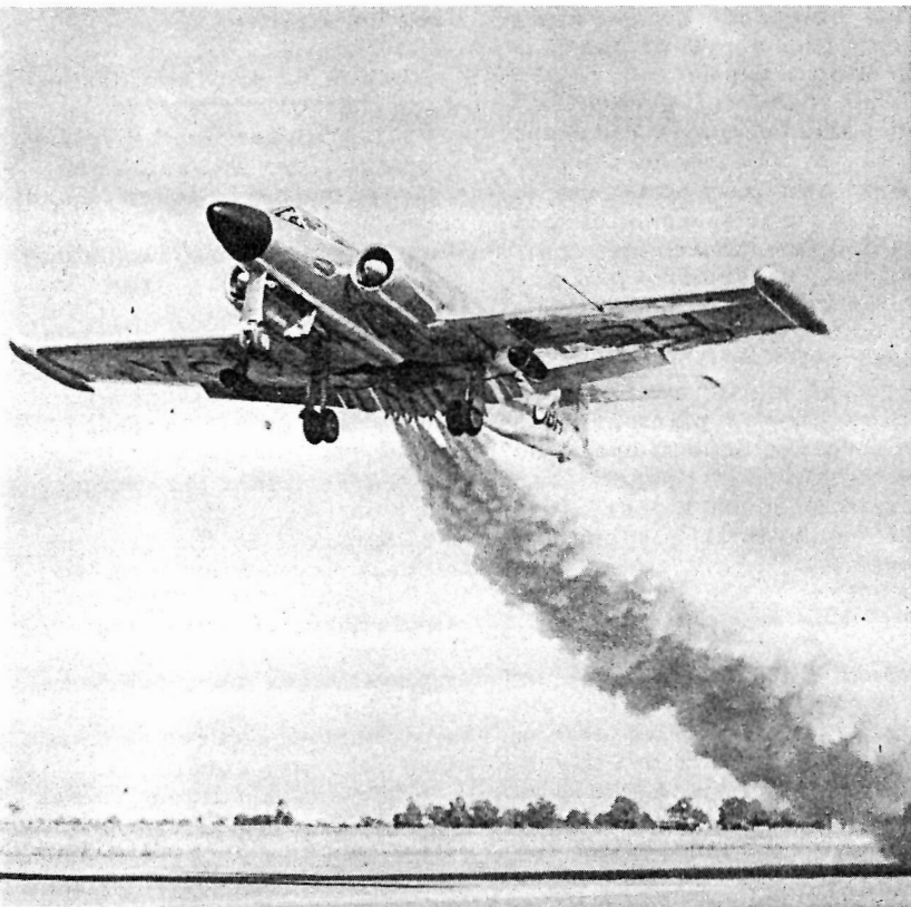
THE CF-100 FIGHTER LEAPS AWAY AS JET-ASSISTED TAKE-OFF BOTTLES HALVE THE NORMAL RUN DURING THE TAKE-OFF TESTS AT THE ROYAL CANADIAN AIR FORCE STATION AT UPLANDS, ONTARIO
