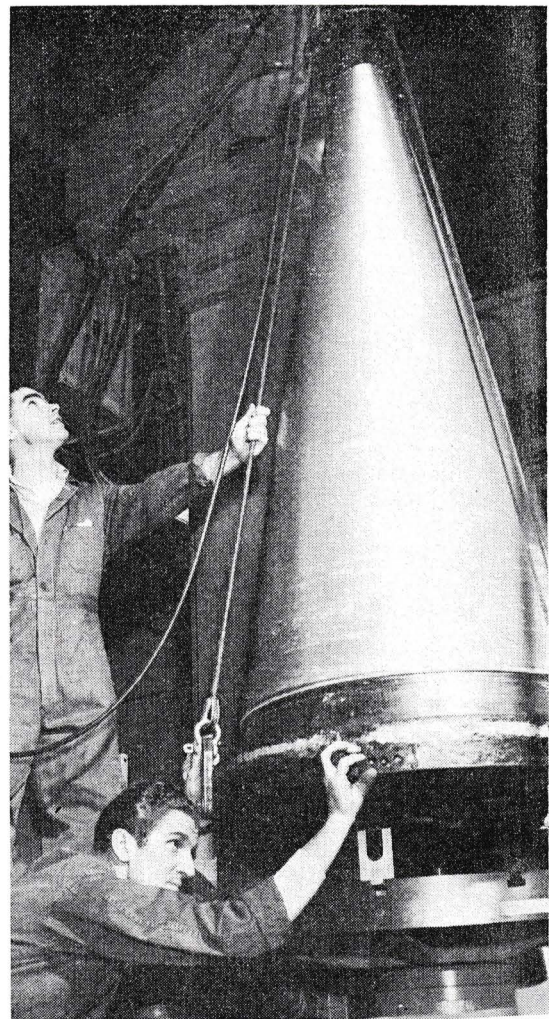
Brunswick of Canada has $500,000 contract to fabricate fibreglass reinforced radomes for the CF-104.
