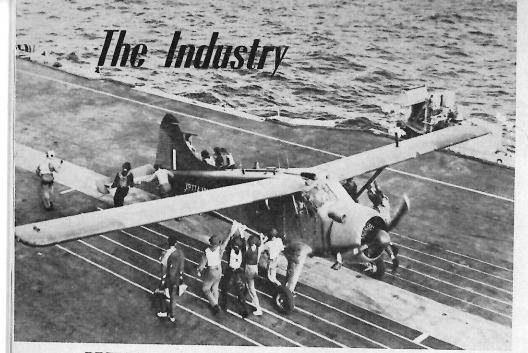
DECK LANDING TRAILS for the Beaver were recently carried out on HMS Centaur by the British Army Air Corps, which acquired 36 DHC-2's last year. Purpose of trials, carried out without usual deck landing aids, was to test feasibility of transporting Beavers to beach-head areas by carrier.
