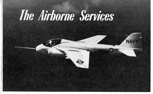
GRUMMAN A2F-1 INTRUDER is being built for the USN as a carrier-based low-level attack bomber with "remarkable" range capabilities. The Intruder is subsonic, and is powered by two Pratt & Whitney J-52's of 8000 lbs. th. each. The crew of two comprises a pilot and a radar operator.
