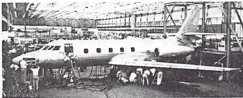
LOCKHEED JETSTAR: Lockheed Aircraft Corp. set an aviation record when they completed a 10-passenger utility jet transport after a development time of only 30 weeks. Built to fill a military transport role, the swept-wing JetStar is powered by two Bristol Orpheus engines mounted in pods attached to the rear fuselage. A second prototype will be powered by four GE J-85's.
