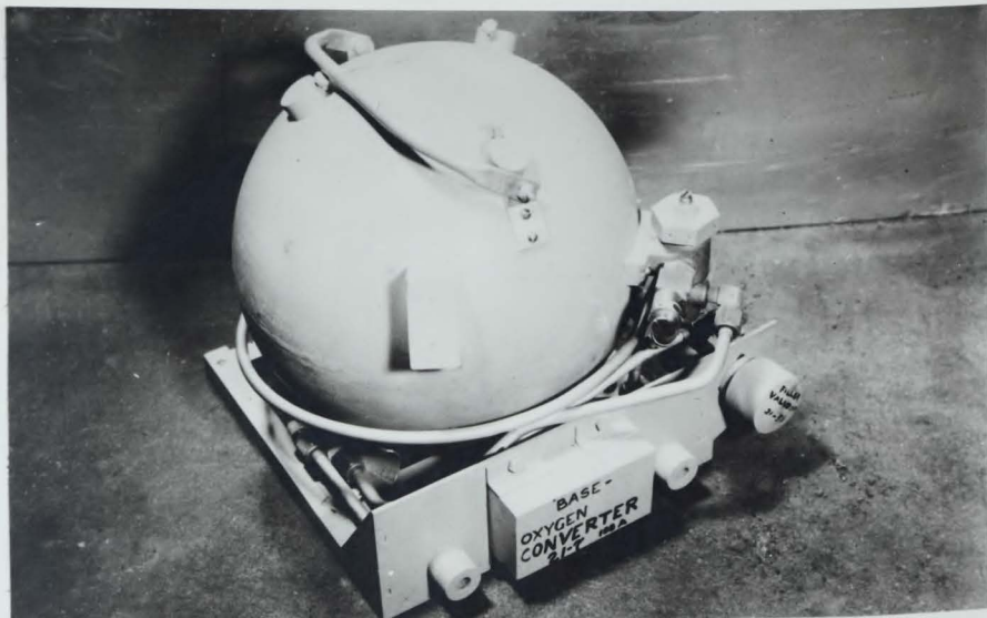
A. 50 LITER LIQUID OXYGEN CONVERTER MOCK UP. \frac{3}{4} VIEW ON FRONT.
