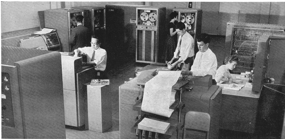
Avro's Computer Capacity was greatly increased with the addition, this year, of the IBM 704 electronic data processing machine shown above. Latest and most powerful digital computer available to industry, Avro's 704 is the only one outside the U.S.
