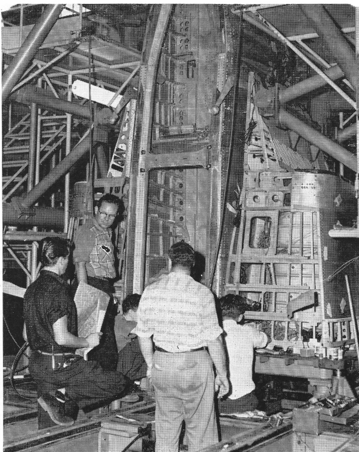
Assembly progress is continually checked against drawings. Here in its jig is the front fuselage section showing both cockpits and engine air intakes.
