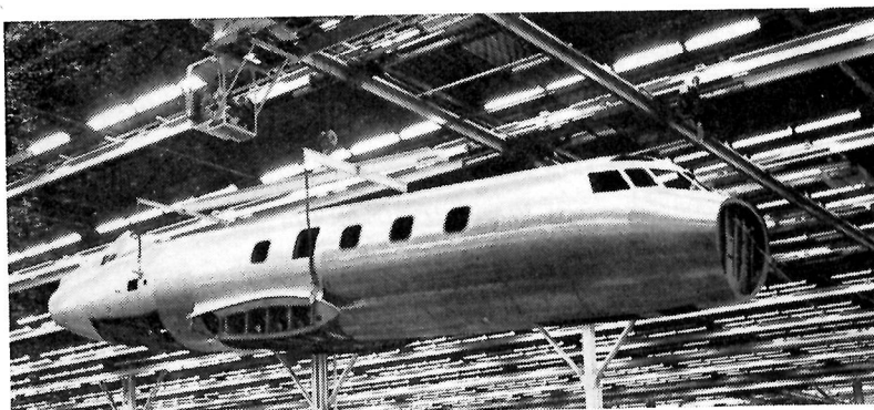
JETSTAR IN ASSEMBLY: First production Lockheed JetStar fuselage is shown being lifted from the main assembly jig and headed for static testing. With exception of nose and pilots' compartment behind forward bulkhead, the entire fuselage is fabricated and assembled in the main jig. First production model of the sleek jet transport is scheduled to fly in July. Cutaway below shows fuselage structural assembly.
