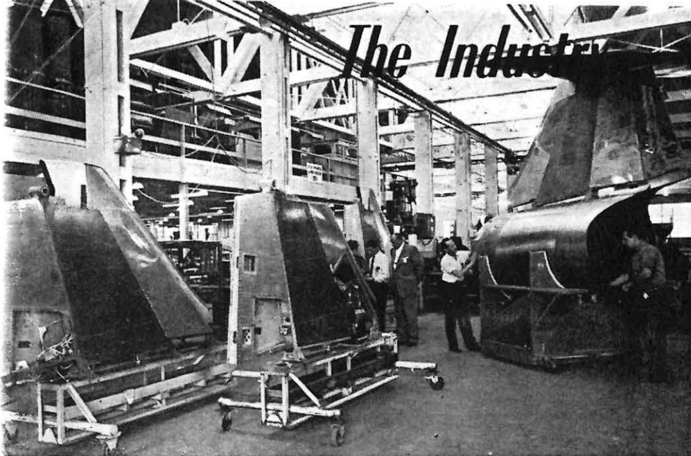
STARFIGHTER PRODUCTION at Canadair Ltd. is in full swing, with components for RCAF CF-104's and the similar F-104G's for Germany, Belgium, Holland and Japan coming steadily from the sub-assembly lines. Scene above is in Plant 2, where rear fuselages, wings and empennages are being produced.
