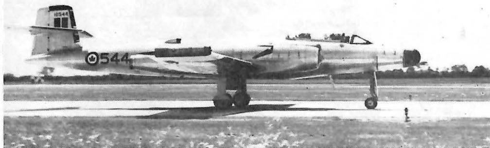
UNIQUE CF-100 was photographed recently taxiing by the passenger terminal building at Malton Airport. The aircraft, a Mk. 5, has a ramjet of unidentified type fitted to each wing tip as well as vortex generators on the wing.
