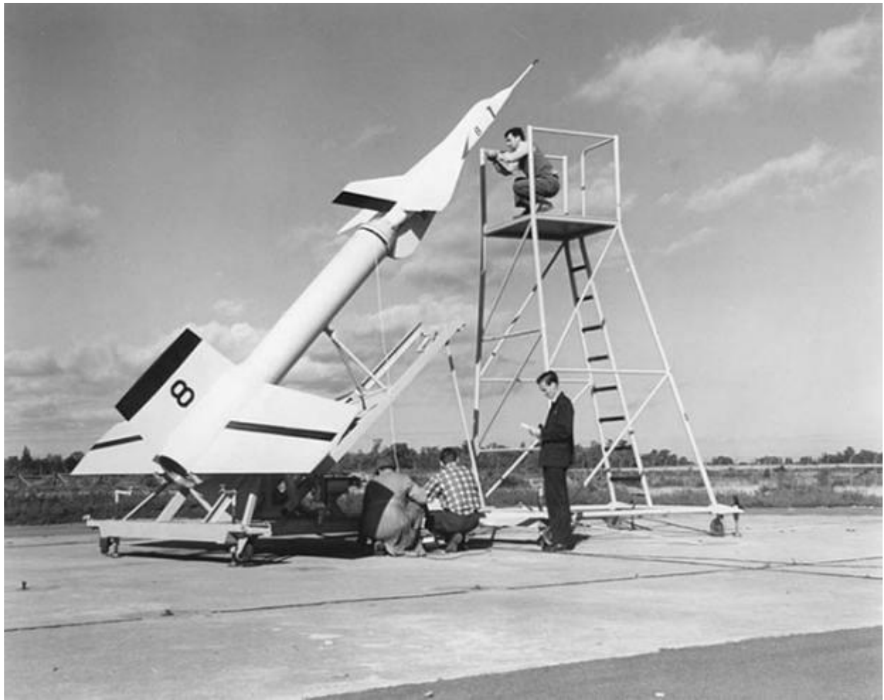
Avro technicians prepare an Avro Arrow test model attached to a Nike booster rocket to fire out over Lake Ontario at Point Petre in the 1950s.
