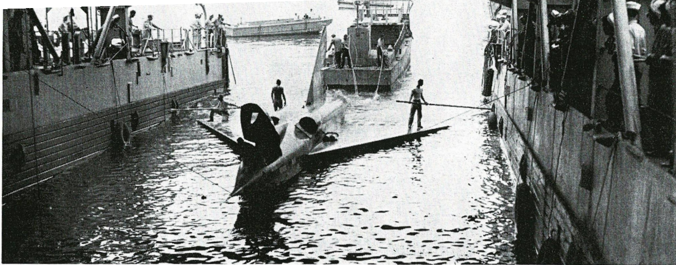
FLOATING into flooded hold of the landing ship-dock, Convair F2Y is guided by lines and poles and then the hold will be pumped out and plane dry-docked.
