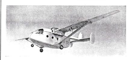
EXTREME ASPECT: H.D.M. 105 experimental light transport aircraft, is being developed jointly by U.K.'s F. G. Miles Ltd., and France's Hurel-Dubois. The H.D.M. 105 consists of a standard Miles M.57 Aerovan fuselage fitted with the Hurel-Dubois all-metal high aspect ratio strutted wing. It is destined to carry out development work towards the H.D.M. 106 "Caravan" transport, and the H.D.M. 107 "Aerojeep".
