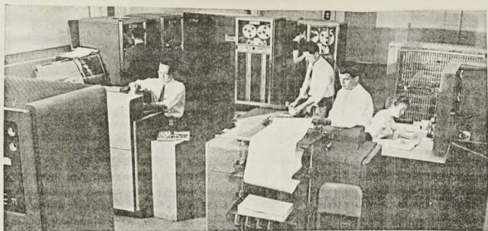
Avro's Computer Capacity was greatly increased with the addition, this year, of the IBM 704 electronic data processing machine shown above. Latest and most powerful digital computer available to industry, Avro's 704 is the only one outside the U.S.
