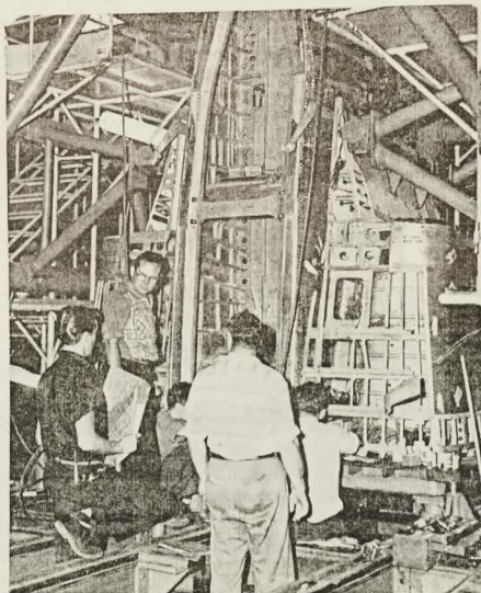
Assembly progress is continually checked against drawings. Here in its jig is the front fuselage section showing both cockpits and engine air intakes.
