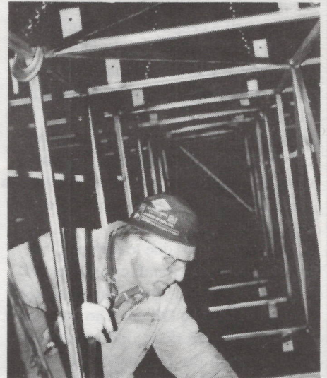
Allan Jackson rubs down part of the frame before applying primer.
