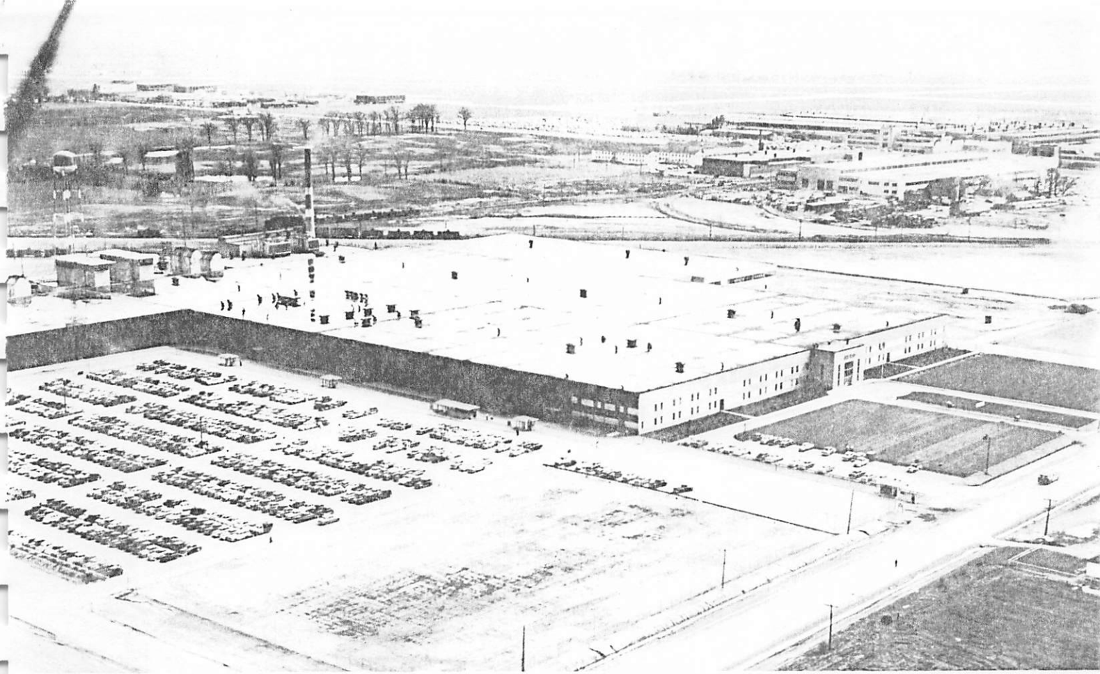
VIEW OF THE GAS TURBINE DEVELOPMENT PLANT
