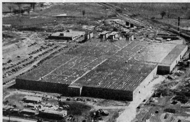
AVRO ORENDA ENGINE PLANT—The new plant with 400,000 sq. ft. of floor area to be devoted to manufacture of Orendas at Malton is almost ready for operation. Most of the machine tools have been installed. Official opening is scheduled for late summer when production should be rolling.
