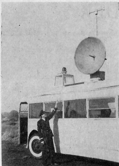
The new one-man radar approach equipment is housed in a bus for mobility.
