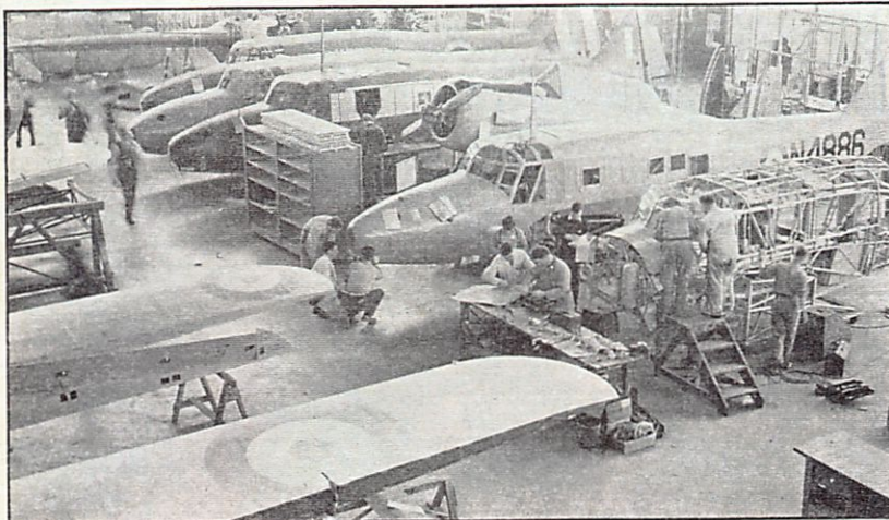
Avro Anson assembly at MacDonald Bros. Aircraft during the war. These aircraft were assembled only at MacDonald; aircraft had been shipped in crates from the U.K. (CAO)
