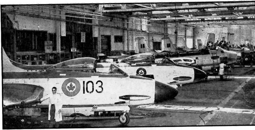
At Eastern Passage, N.S., Fairey of Canada specializes in the maintenance, repair and overhaul, and modification of naval aircraft for the RCN, and maritime aircraft for the RCAF. Above, a line of Banshees; below, Neptune after overhaul and modification.
