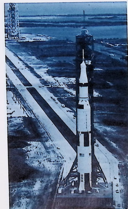
The Space Vehicle for Apollo 11 is rolled out of the Vehicle Assembly Building down the 3.5 mile Crawlerway to Launch Complex 39-A at a speed of one mile per hour.
