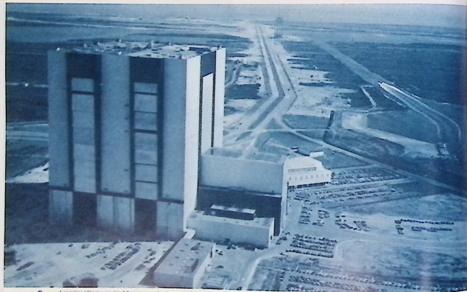
Four Apollo/Saturn V Moon rockets, each towering 363 feet, can be assembled at once in one of the largest—by volume—buildings in the world, the Vehicle Assembly Building (VAB).
