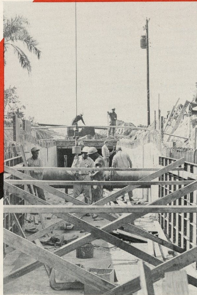
Box Culvert construction on 49th Street South
