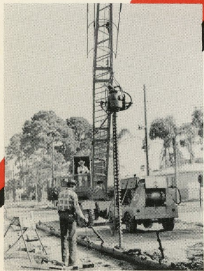
49th Street Storm Drainage Project
