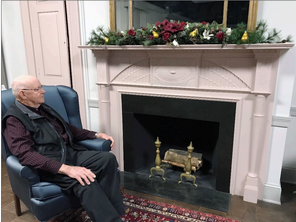
Figure 14 Photograph of the mantel and cupboard provided by the HSCC and showing the current paint finishes. The level of detail evident in the profiled ornament is evidence of the few extant paint layers.
