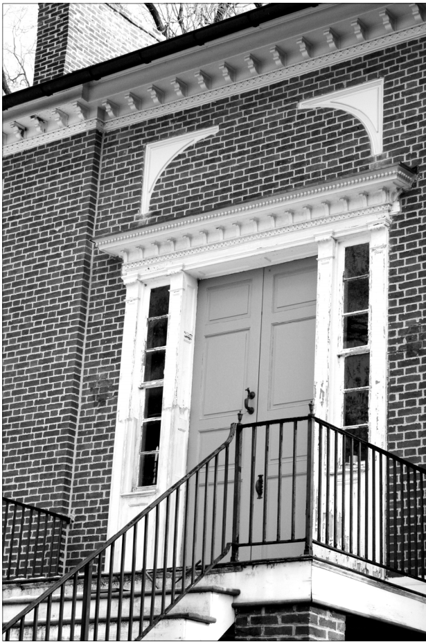
Figure 4: Doorway on the principal story with narrow pilasters flanking the sidelights and an elaborate cornice. Note the wood panels above the door, the roof cornice, and the Flemish bond brickwork. Photograph by Cathy Baty.
