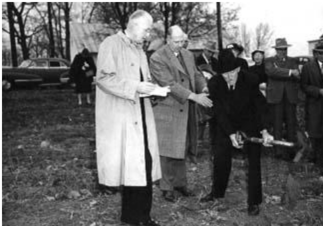
Several members of Trinity Lutheran Church, host of Dutch Picnic, near Smallwood participated in groundbreaking for a new church on April 17, 1955. From left to right: Rev. W. Harold Redcay, Harvey Bitzel and Charles Niner. Mr. Niner was one of three 1951 Dutch Picnic attendees who had attended every event since 1877. Historical Society of Carroll County collection, gift of Gladys Wimert, 1955.
