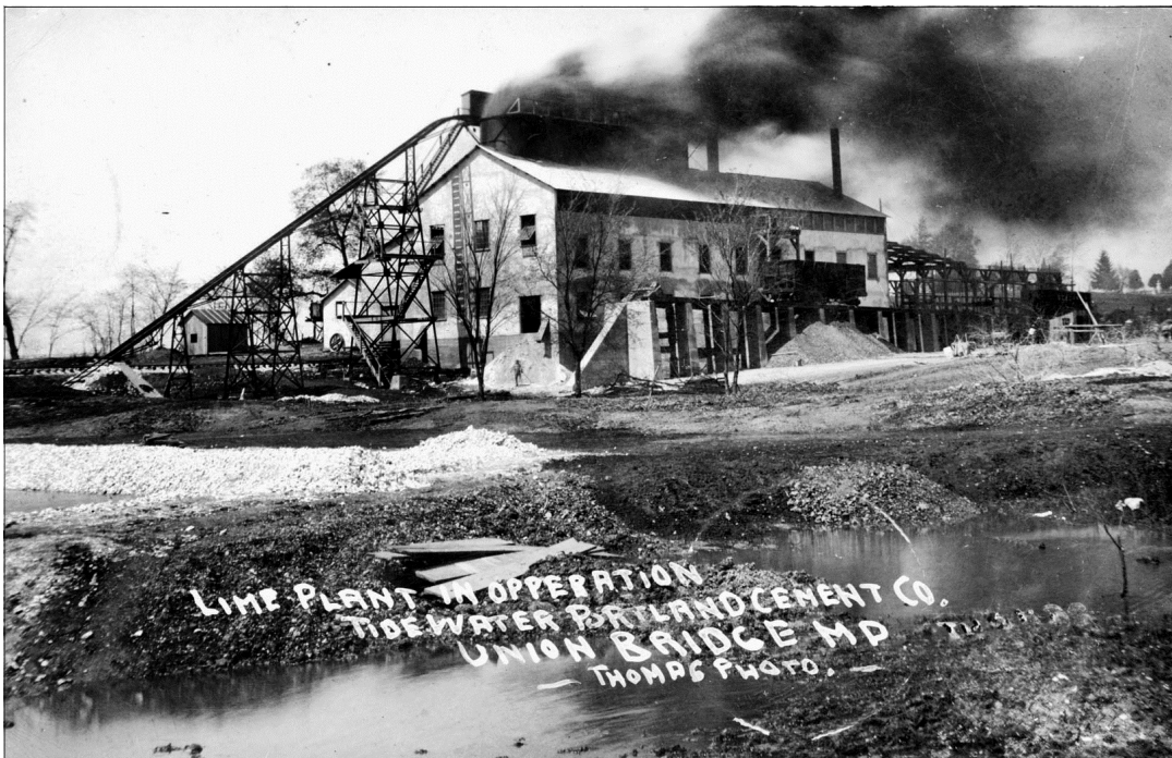
Tidewater's hydrated lime plant, completed in the spring of 1910, showered Union Bridge with lime dust for a year before the rest of the buildings were finished. Photograph by Frank S. Thomas.
