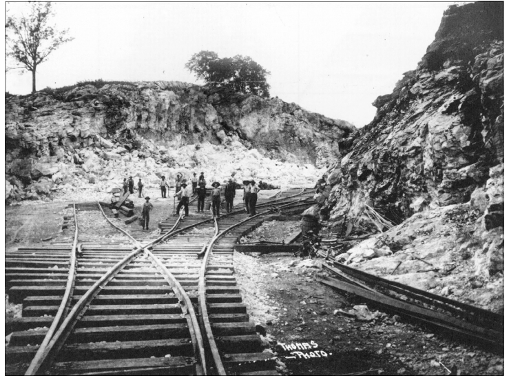
Laying track in a Tidewater quarry in 1918. Limestone was loaded into small cars called "dinkeys" and hauled by locomotive to the crusher building. Photograph by Frank S. Thomas. Courtesy of Lehigh Heidelberg Cement.
