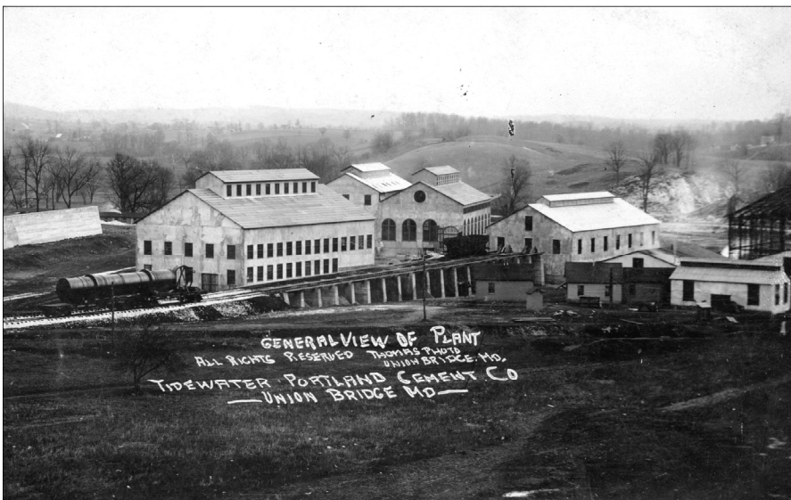
This early 1911 photo shows the partially completed Tidewater cement plant. More buildings were added before cement production began. One quarry appears on the right. Photograph by Frank S. Thomas. Courtesy of Angelo Monteleone.
