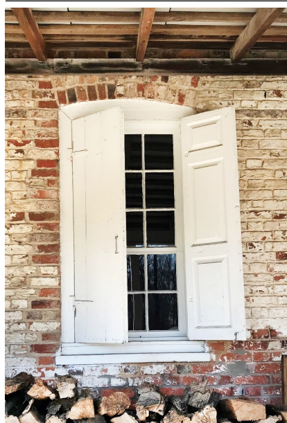
Window with wooden header and shutters with hand-forged hinges. (HSCC photo, 2023)
