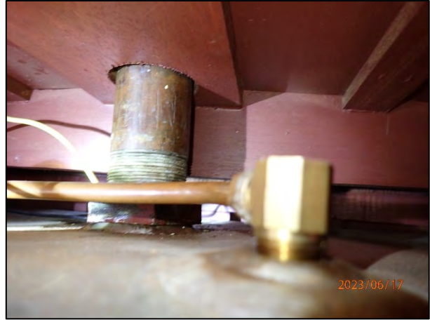
Fill Pipe And Vent Tube
