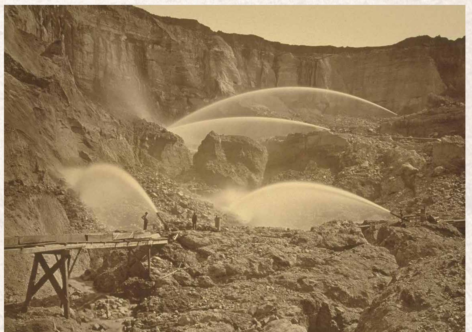
Hydraulic mining at the Malakoff Diggings, Nevada County, California. UC Berkeley, Bancroft Library. BANC PIC 1905.17175:099--ffALB.
