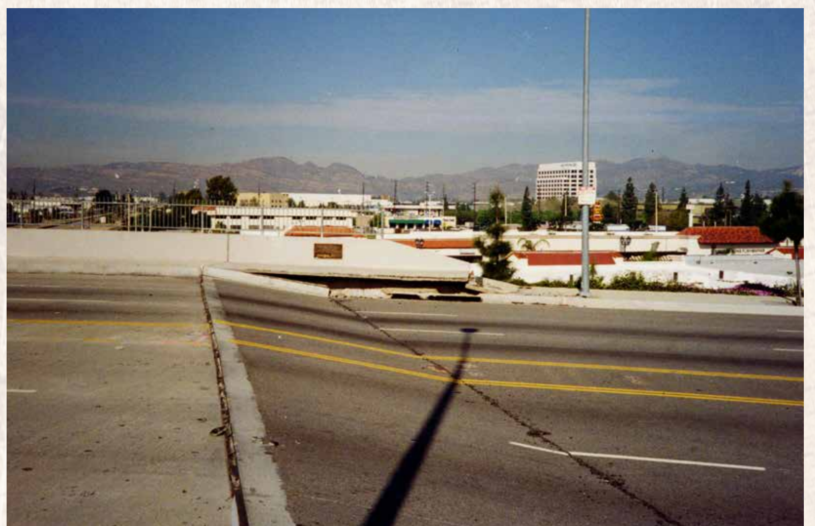
Photo of damage to Nordhoff Way overpass over the railroad tracks east of Corbin Ave. Photograph by Kris Tacsik and Michael Swift. California State University Northridge. University Library. Map Collection. NEPCo37.
