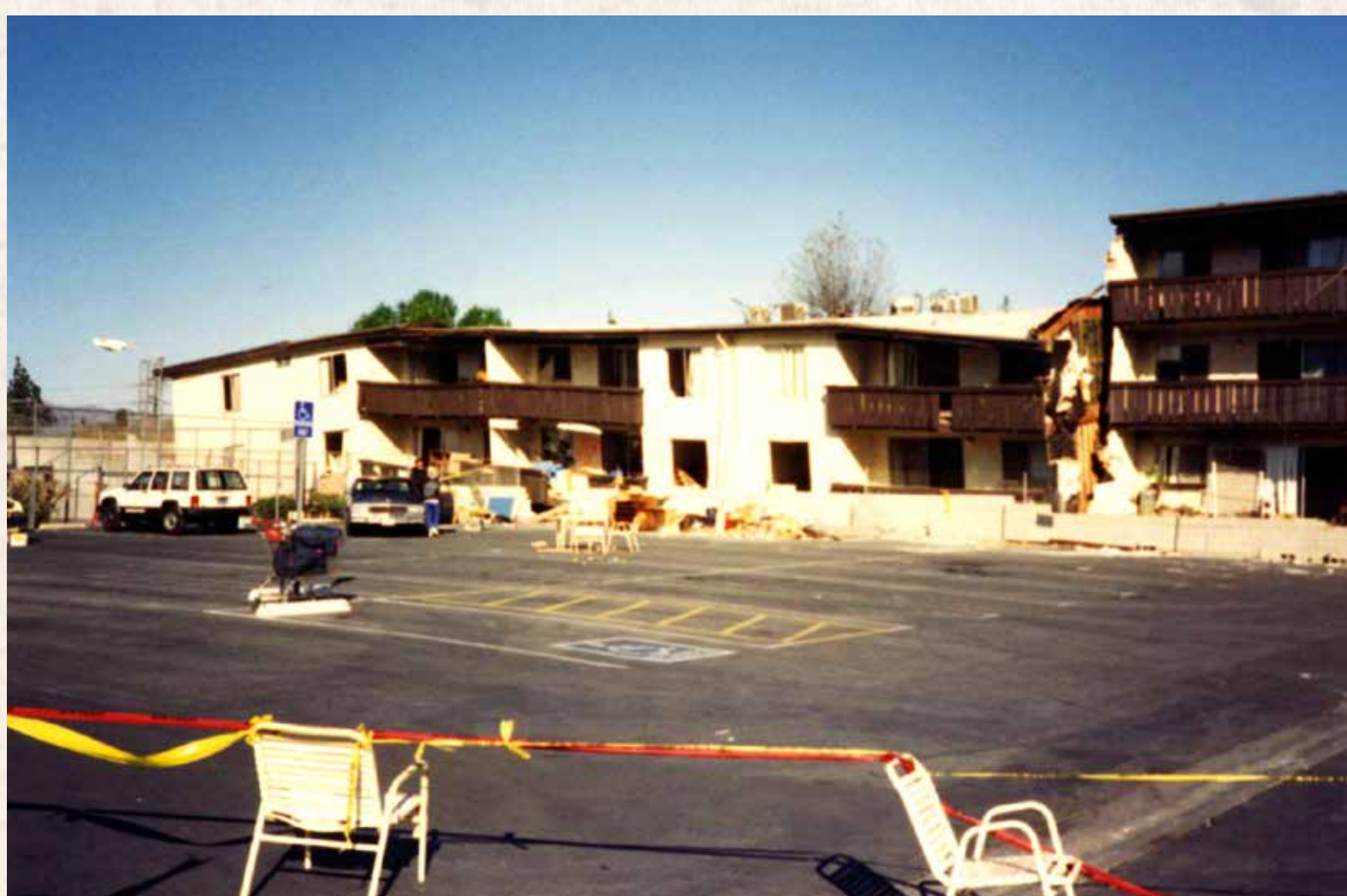
The rear parking lot behind the Northridge Meadows Apartment Complex. The first floor of the three-story structure completely collapsed, resulting in the largest concentration of deaths in the Northridge earthquake. Photograph by Kris Tacsik and Michael Swift. California State University Northridge. University Library. Map Collection. NEPCo94.
