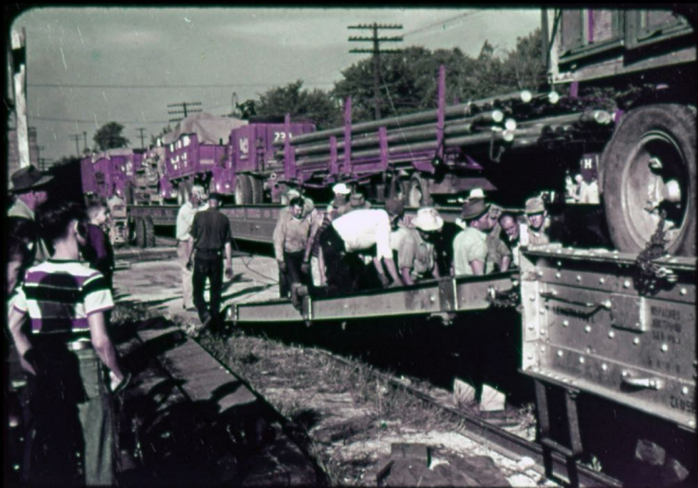
Cook house, menagerie, and heavy equipment arrive first.
