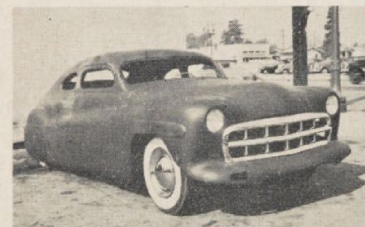
AYALA-made '41 Ford Business Coupe has '42 Ford fenders, with fadeaways added. Six-inch cut in top, with windshield area expanded into top three inches. Hood is made from flat stock
