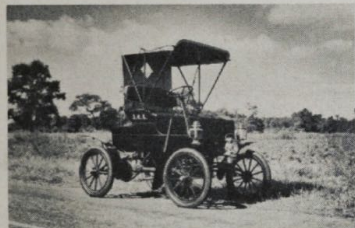
EARLY 1908 model Jewell with its distinctive piano-box style body. What would correspond to the keyboard section of a piano is the section behind the seat in which the one-cylinder engine is housed.
