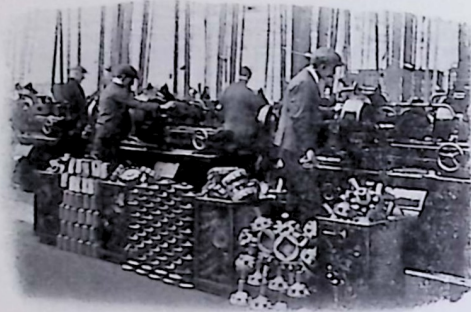
View in Machine Shop.
