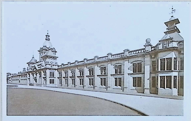
ADMINISTRATION BUILDINGS, ALEXANDRIA
